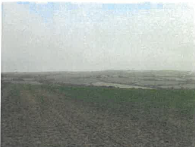
Distant view (left) of the 16ha (Band D) solar farm at Treswarrow Farm
