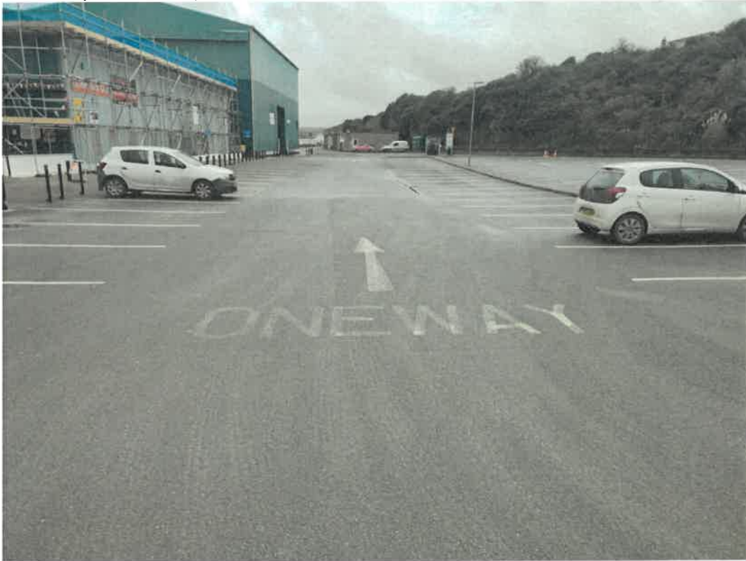
16. One way / no entry markings - re-done.
