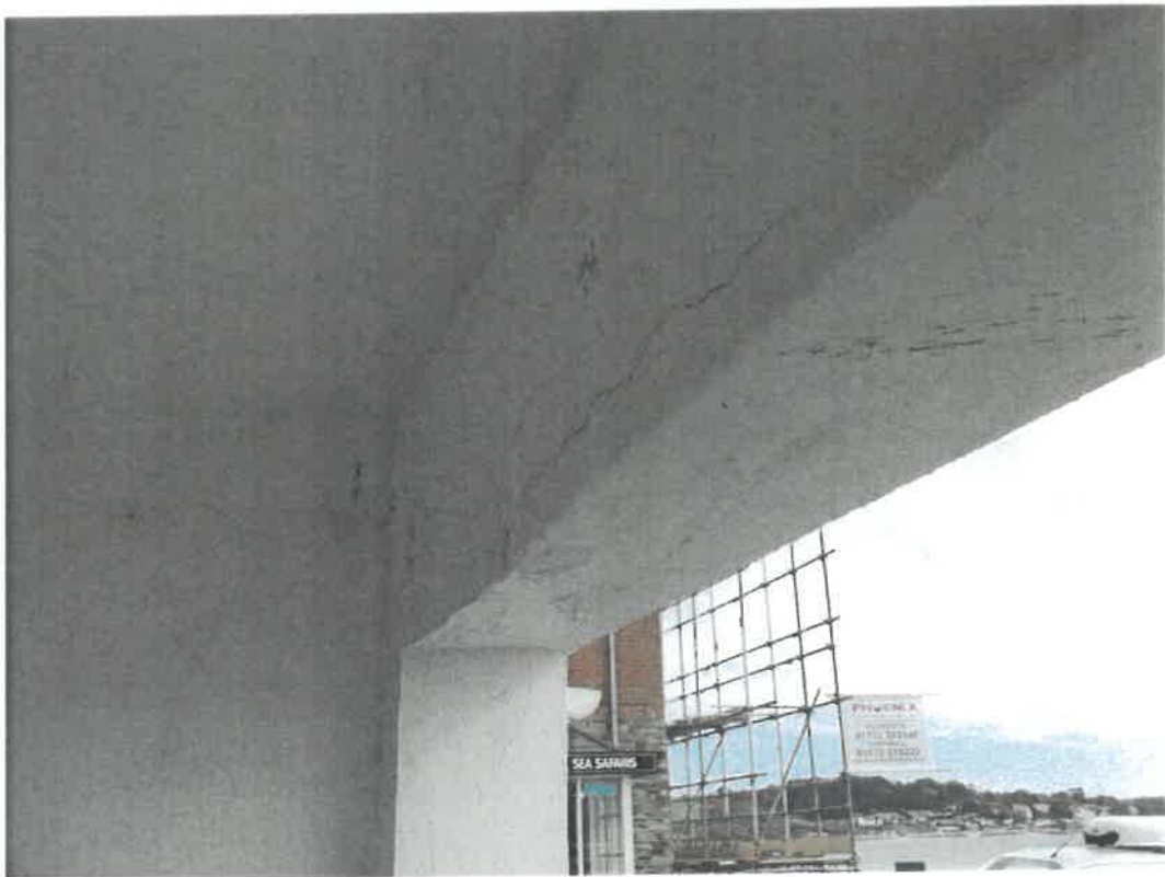
Photo 4 - Cracking evident to lintel area
