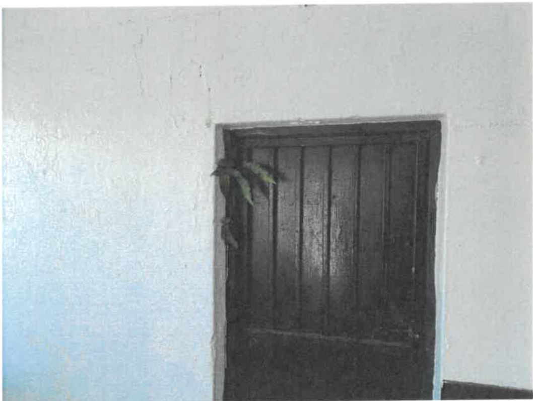
Photo 6 - General decay to internal plaster finish
