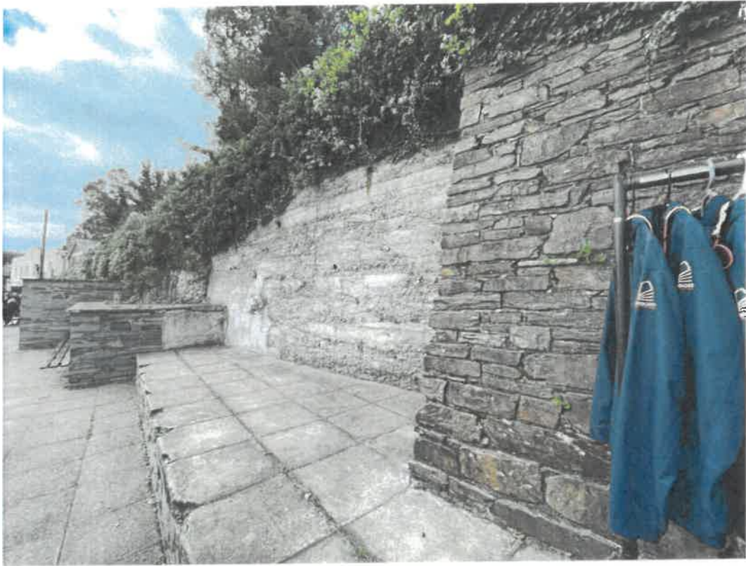
Photo 4 - Settlement of slabs at high level
