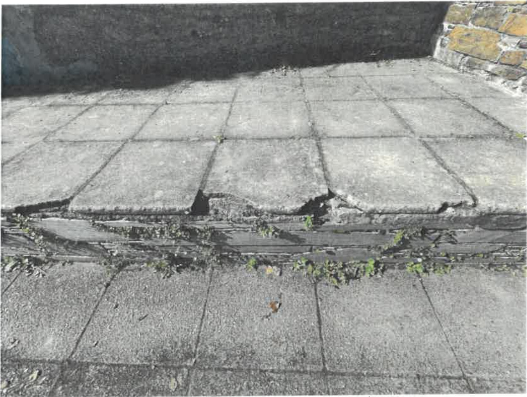
Photo 2 - Missing areas of stone bank need infilling
