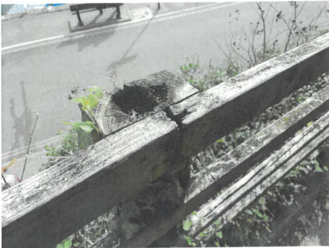
Photo 6 – Timber post and rail fence with evidence of decay and wet rot attack
