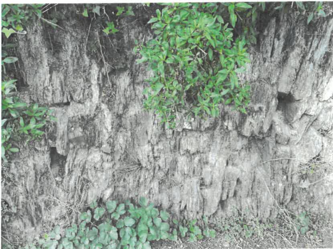
Photo 2 - Missing areas of stone bank need infilling
