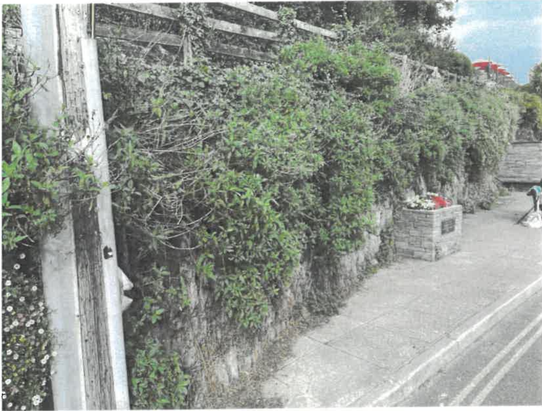
Photo 6 – Timber post and rail fence with evidence of decay and wet rot attack
